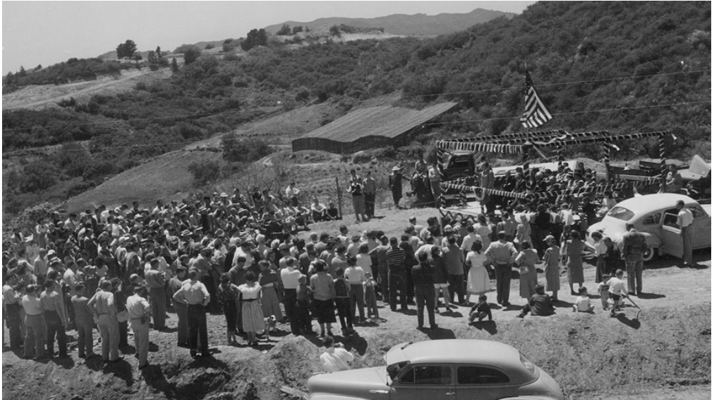
Crestwood Hills groundbreaking with a plant nursery in the background.
